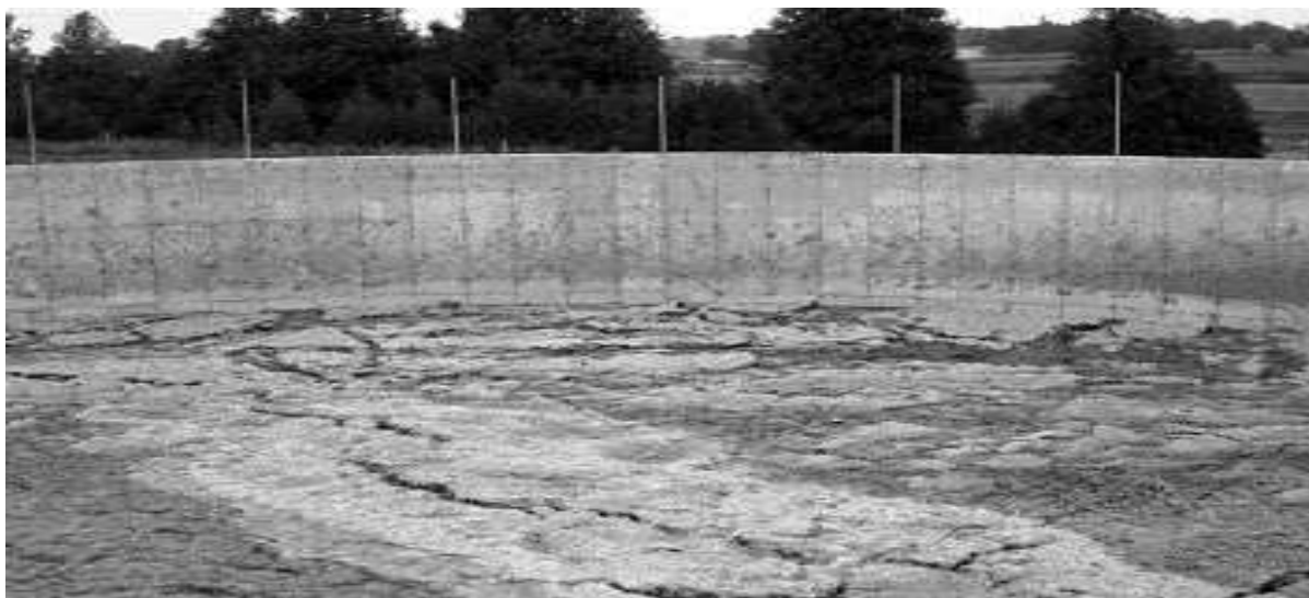
Figure 5.3: Crust Formation on a Liquid Manure Storage
